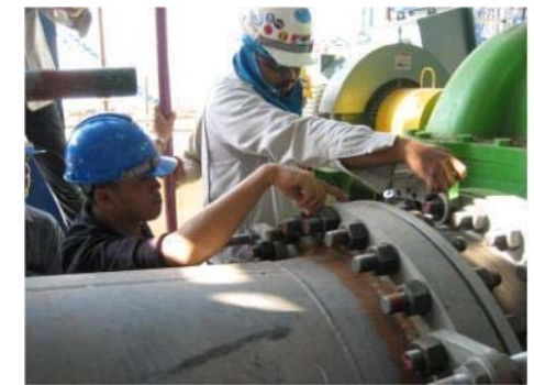
Hydraulic Bolt Torque MC (5 sets)
